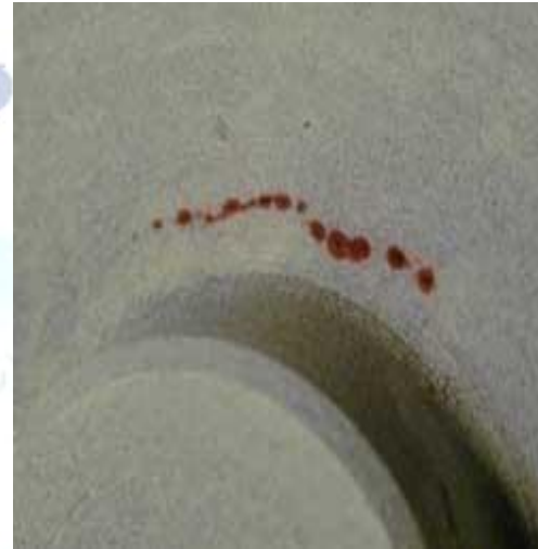
Fig-9: Defects for LPT
