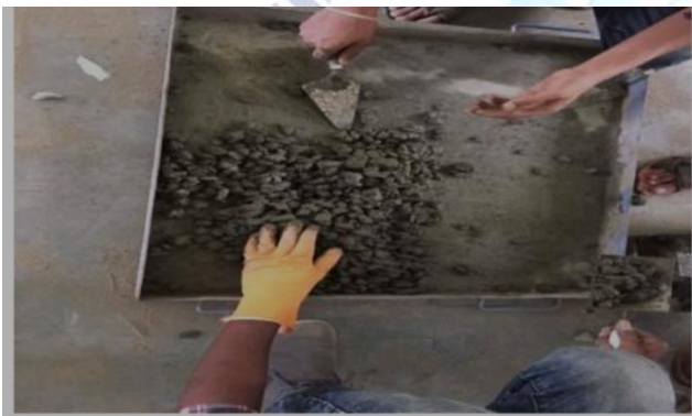
Mixing of pervious concrete
