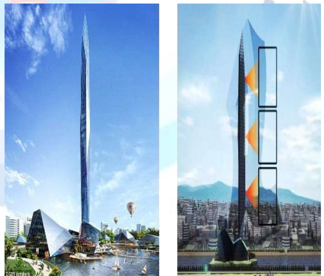
Fig 7: Infinity Tower (under construction in South Korea)
