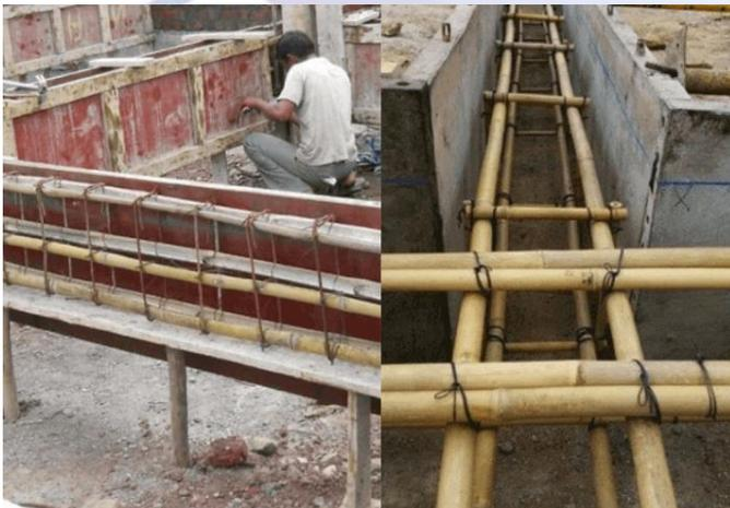
Moreover, BFRC exhibits improved resistance to shrinkage cracking and thermal cracking compared to conventional concrete. The incorporation of bamboo
