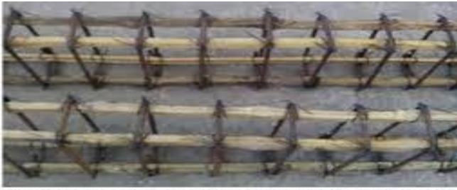
Fig. 1: Bamboo as a reinforcement in column [11]
