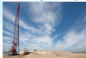
Fig:11 Vibro Compaction
