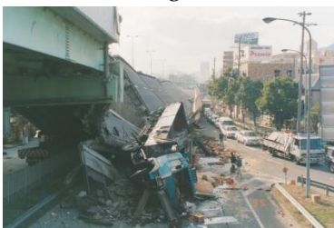
Fig:1 Nishinomiyama Bridge 1995 Kobe earthquake, Japan Soil liquefaction occurs most frequently in sandy, silt-laden, gravel-based, loose or poorly drained soils. Quicksand is an example of this phenomenon. The
