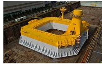
Fig :6 Ideol's 2MW floating wind turbine installed off France
