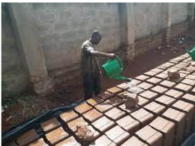
**Fig: Manual curing**
