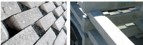
Fig. precast concrete crib retaining wall
