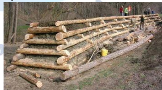
Fig: Wooden log crib wall
