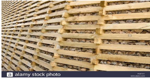
Fig. Timber crib retaining wall
